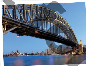
Sydney Harbor Bridge
