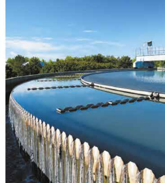
C | Water, with fewer solids suspended in it, pours from the surface of a settlement pond. This water still contains dispersed and dissolved solids.
