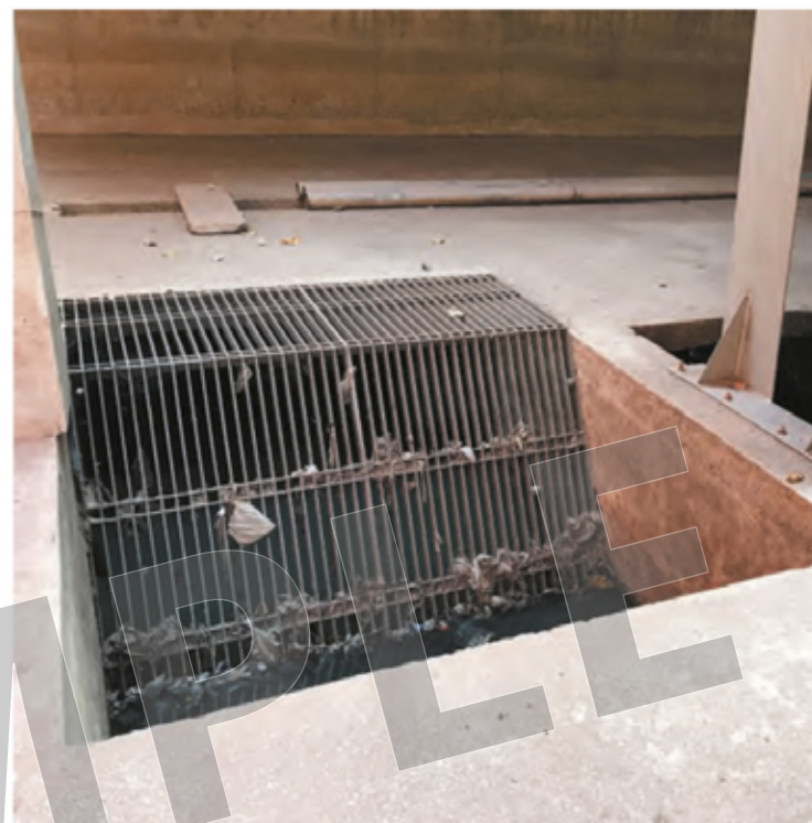
A | Waste water from homes, offices and street drains contains large solids such as leaves, rubbish and lumps of human waste, as well as smaller solids. In the first stage of treatment, waste water passes through a screen, which acts as a sieve .
