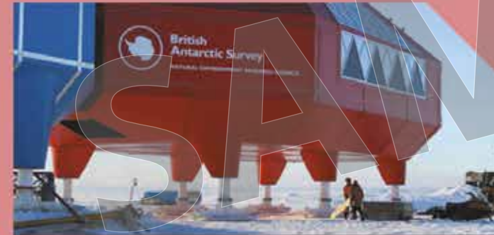
B | This is Halley station in Antarctica. The snow here never melts. To prevent the station from becoming buried, the buildings can be raised higher each year.
