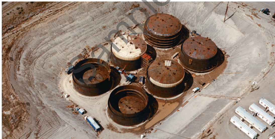
◀ Storage tanks at Hanford, Washington, contain 200 million litres of high-level nuclear waste. Each tank pictured here holds 4 million litres.
