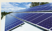
FIGURE 7.4.13 Solar panels are used to convert sunlight into electrical energy using the photoelectric effect. Scientists hope to improve this in order to make solar cells an economic alternative to fossil fuels for large-scale energy generation. One approach includes research on other semiconductors that absorb light more efficiently.
