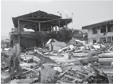
This photograph shows buildings that were damaged by the 2004 tsunami in Aceh, Indonesia.
