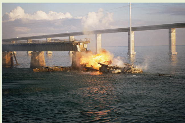
FIGURE 2.5.3 An old bridge is demolished with the help of explosives.
