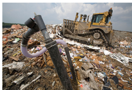
FIGURE 2.2.12 Pipes buried in this rubbish tip collect biogas.
