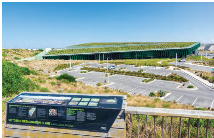
FIGURE 6.11.1 The Victorian Desalination plant, Wonthaggi, Victoria.
