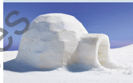
FIGURE 2.2.4 Air pockets in compressed snow enable igloos to keep their occupants warm relative to outside temperatures.
