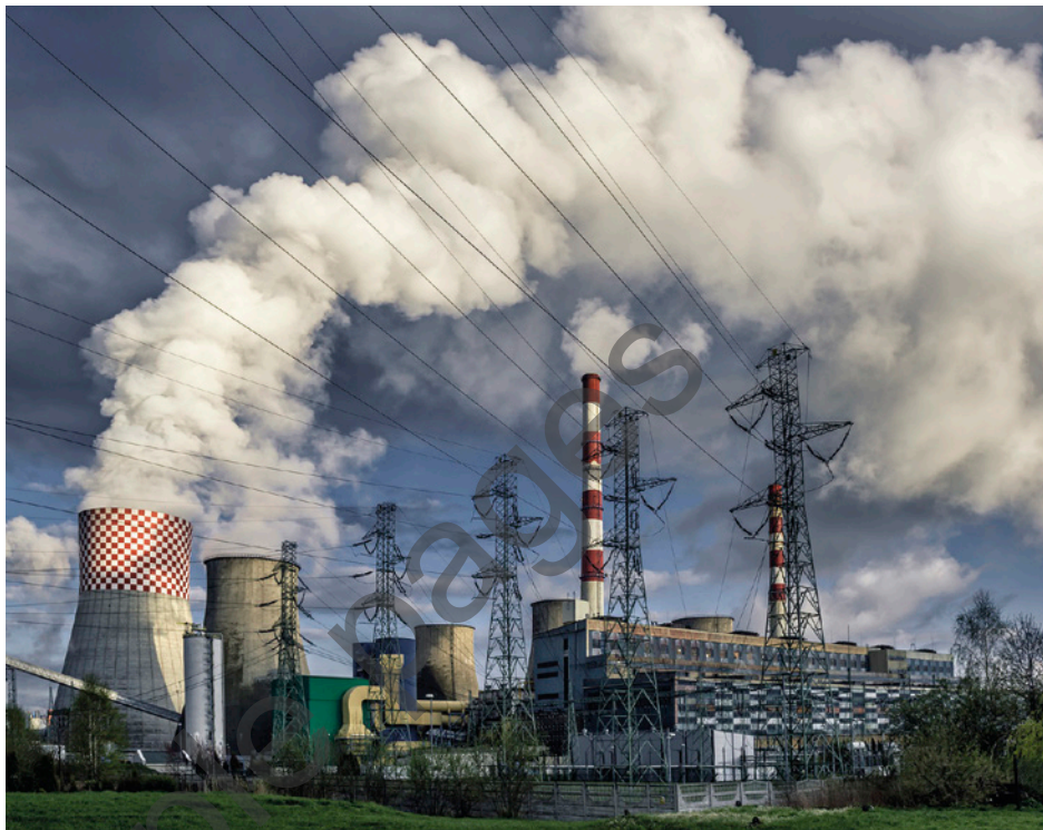
FIGURE 2.1.1 Most power plants use thermal energy to produce steam. That steam does work turning turbines, which generate electricity.
