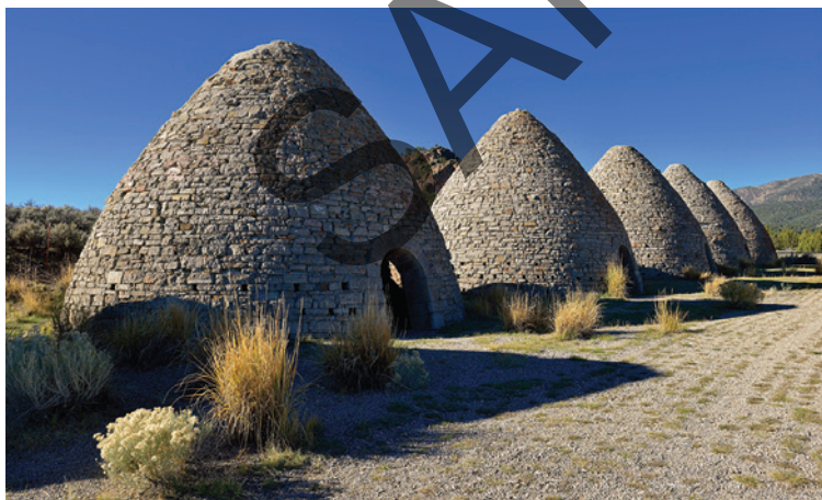
FIGURE 3.5.15 These ovens in Nevada, USA, were built between 1876 to 1879 to make charcoal.
