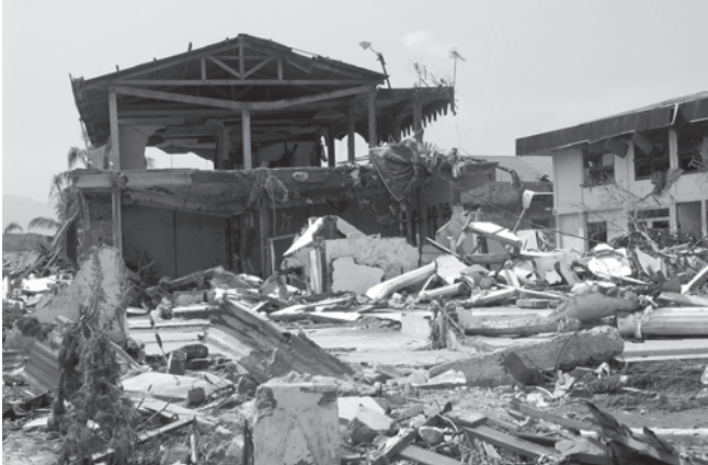
1.3.1 Buildings damaged by the 2004 tsunami in Aceh, Indonesia
