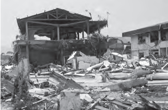
1.5 Buildings damaged by the 2004 tsunami in Aceh, Indonesia
