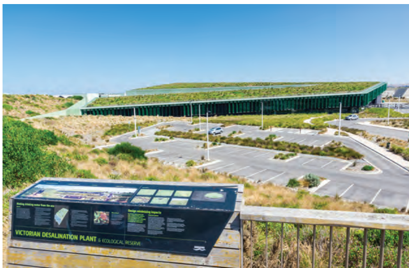
FIGURE 6.11.1 The Victorian Desalination plant, Wonthaggi, Victoria.
